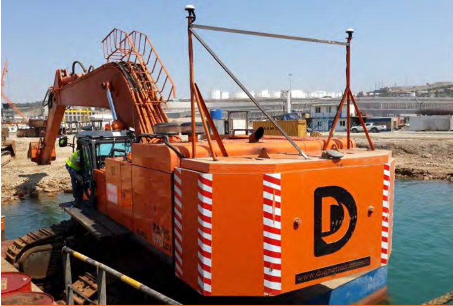
Overview of Excavator
